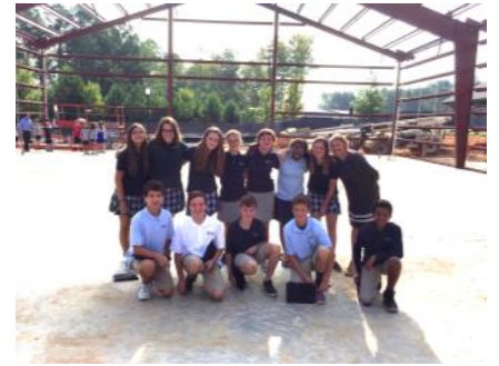
Each class at PES will have the opportunity to leave their “mark” on the new building. Pictured is the 8th Grade after signing the steel.
